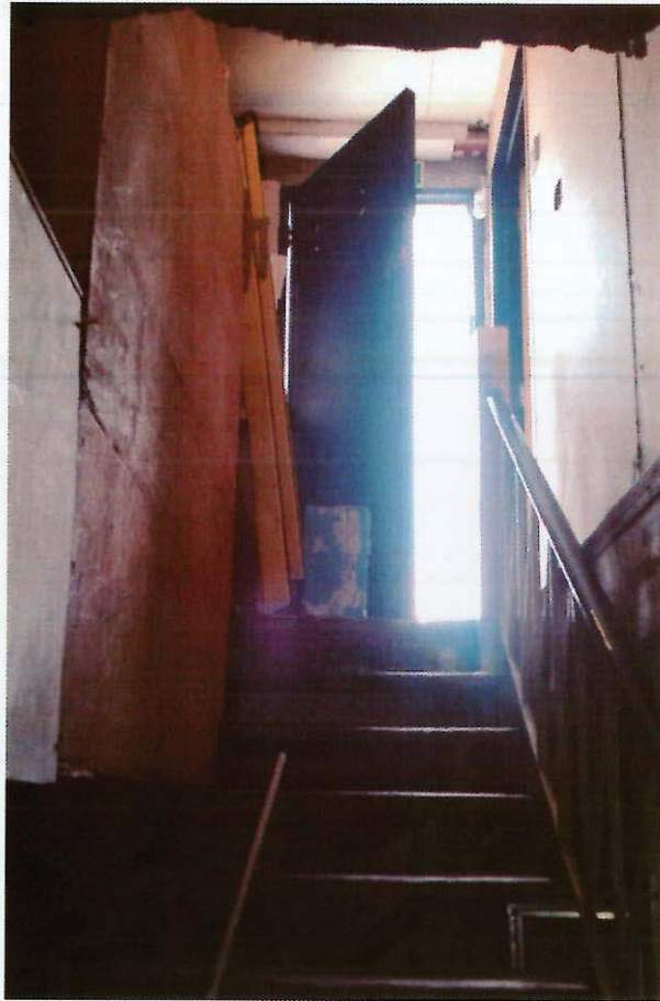
15. Basement – Looking up the stairs leading from the basement towards fire exit.
