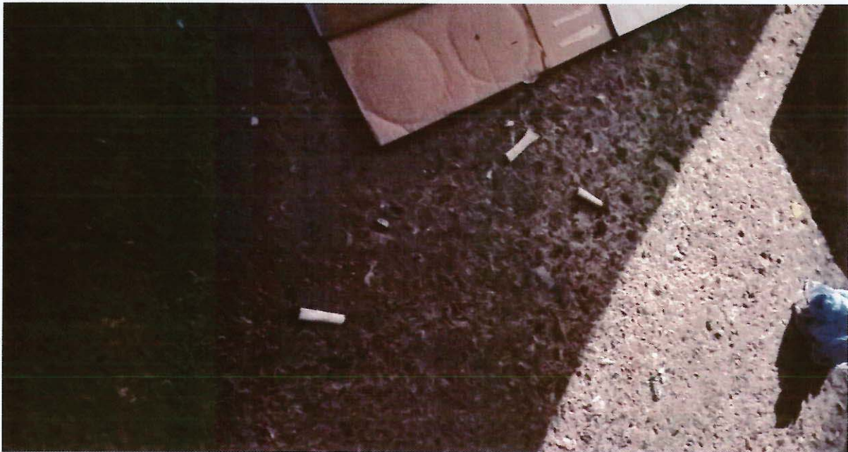
16. The floor of the basement showing discarded cigarettes near to the pile of cardboard boxes shown in image 14.
